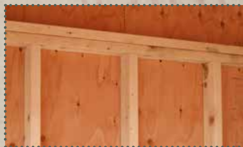
Double Plated Wall Header
